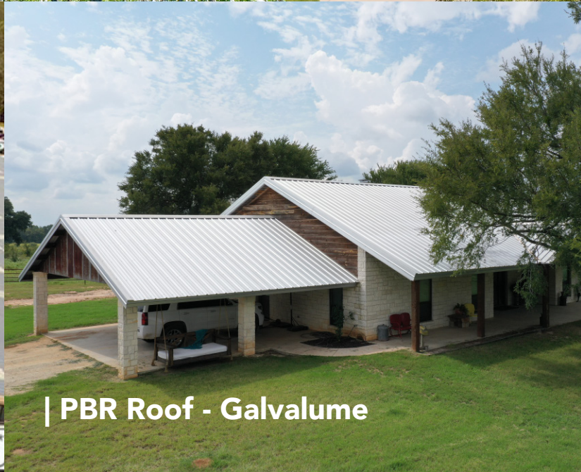
| Commercial PBR Roof - Galvalume w/Skylights
