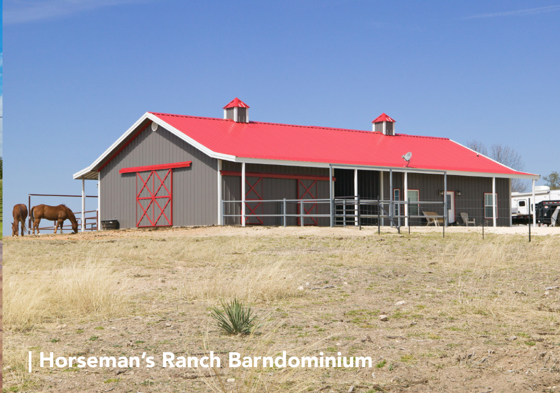
| Thurman Roofing And Construction Shop with Apartment
